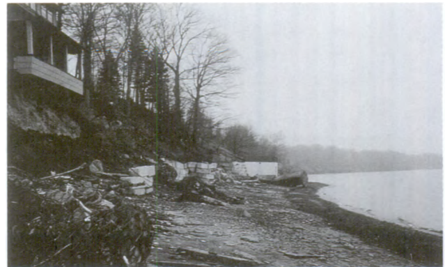
Erosion of bluffs overlooking the Great Lakes has caused an immediate hazard to many lakefront homes. Some were certified as being in danger of imminent collapse and were eligible for federal assistance under Upton-Jones to be relocated.
