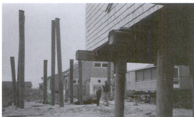
Piles are generally made of wood or prestressed concrete. They often are braced against lateral and shear forces using wood knee and cross bracing, steel rods, and guy wires.
