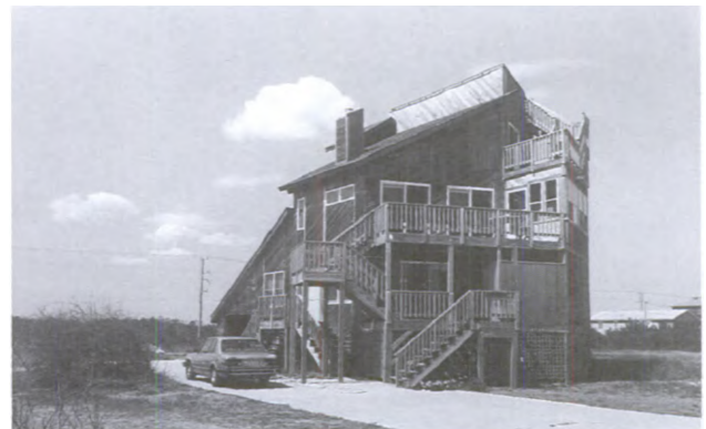
This multistory home in Nags Head, North Carolina, was relocated from an oceanfront VE Zone to an AE Zone.
