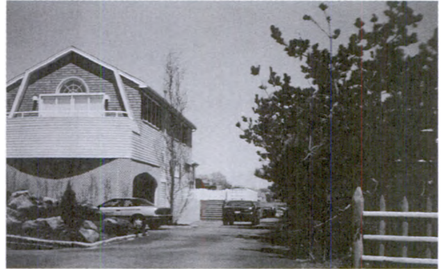
The elevation of this home resulted in the elimination of $25,000 annually in repetitive flood insurance claims. Plantings and berms disguise the retrofit and enhance the landscape.
