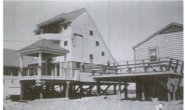
Residences are typically elevated on pressure-treated, cross-braced wood piles. One local contractor constructs over 25 residential elevation projects a year.
