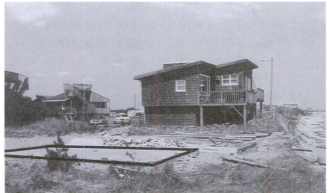
Many jurisdictions require that the old lot be returned to pristine conditions or its natural state. Note the concrete slab and construction materials that must be removed. Some of these lots have remained private property, while others have been utilized for public access to waterfront areas.
