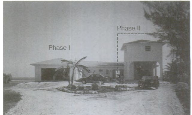
The addition was constructed to withstand expected storm events. If substantially damaged, the original home would have to be reconstructed in compliance with NFIP requirements.
