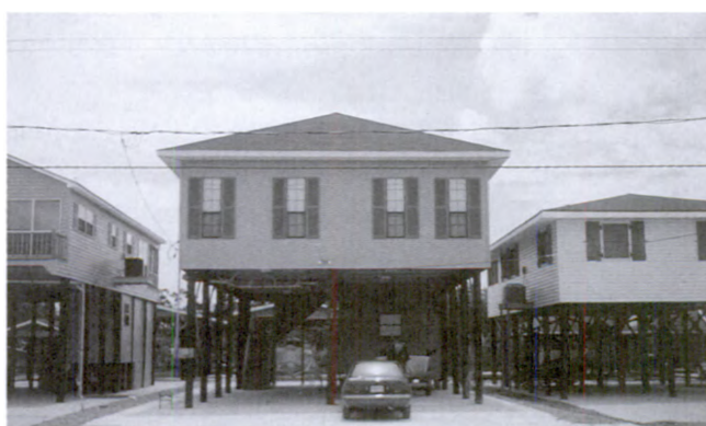
The home is set on the new pile foundation system.
