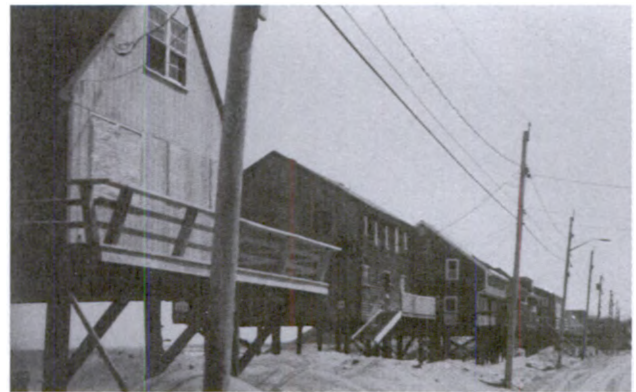
Many homes in Sandwich, Massachusetts, were relocated landward on their existing lots after severe dune erosion from an October 1991 Northeaster.
