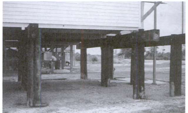
Each pair of piles is connected with bolts.
