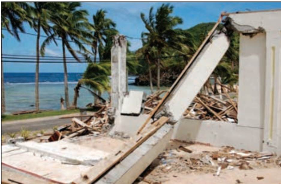
Figure 3-12. Damage from the 2009 tsunami (Amanave, American Samoa)
