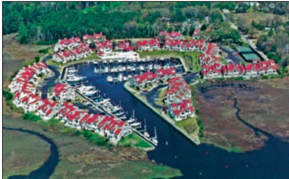
Figure 4-10. Example of parcels difficult to develop (mixed-use marina/ townhouse development)
