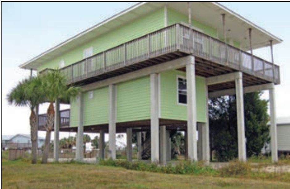
Figure 2-23. Above-grade enclosure (Perry, FL)
