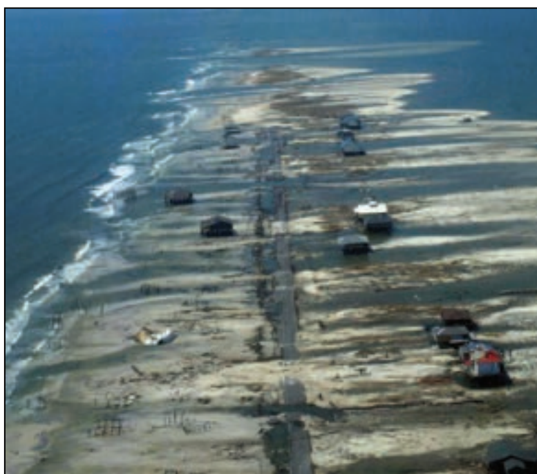
Figure 4-16. Narrow, low-lying areas and barrier islands (such as Dauphin Island, AL, shown in the photograph) are routinely subjected to coastal storm effects (Hurricane Katrina, 2005) SOURCE: USGS
