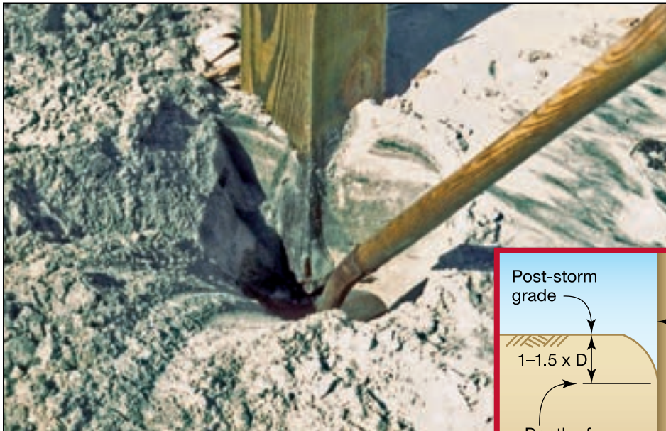
Figure 3-48. Determination of localized scour from changes in sand color, texture, and bedding (Hurricane Fran, 1996)
