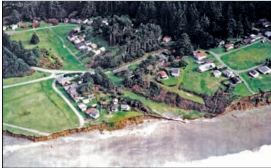
Figure 4-19. As buildings in this Humbolt County, CA, community are threatened by bluff erosion along the Pacific Ocean, they are moved to other sites on the jointly owned parcel
