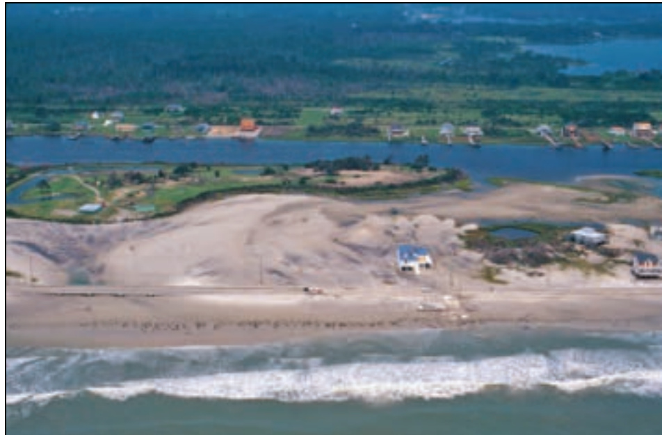
Figure 3-34. Overwash on Topsail Island, NC, after Hurricane Bonnie in 1998 SOURCE: USGS
