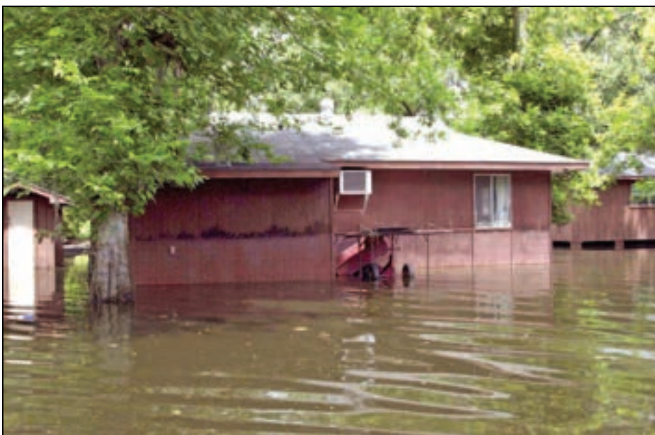
Figure 3-4. Storm surge flooded this home in Ascension Parish, LA (Tropical Storm Allison, 2001)
