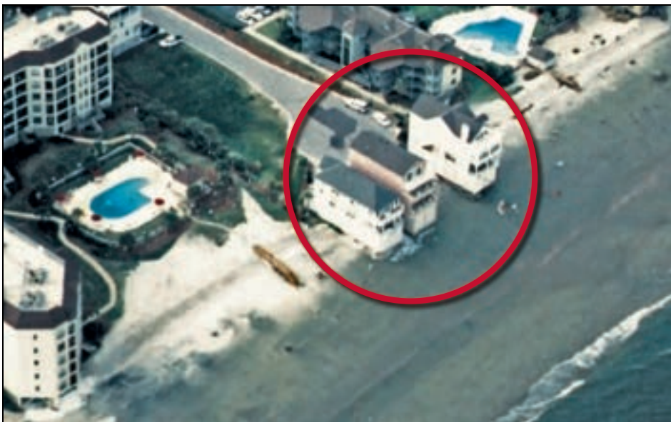
Figure 4-20. Three 2-year-old South Carolina houses left standing on the beach as a result of rapid erosion associated with a nearby tidal inlet (July 1997)
