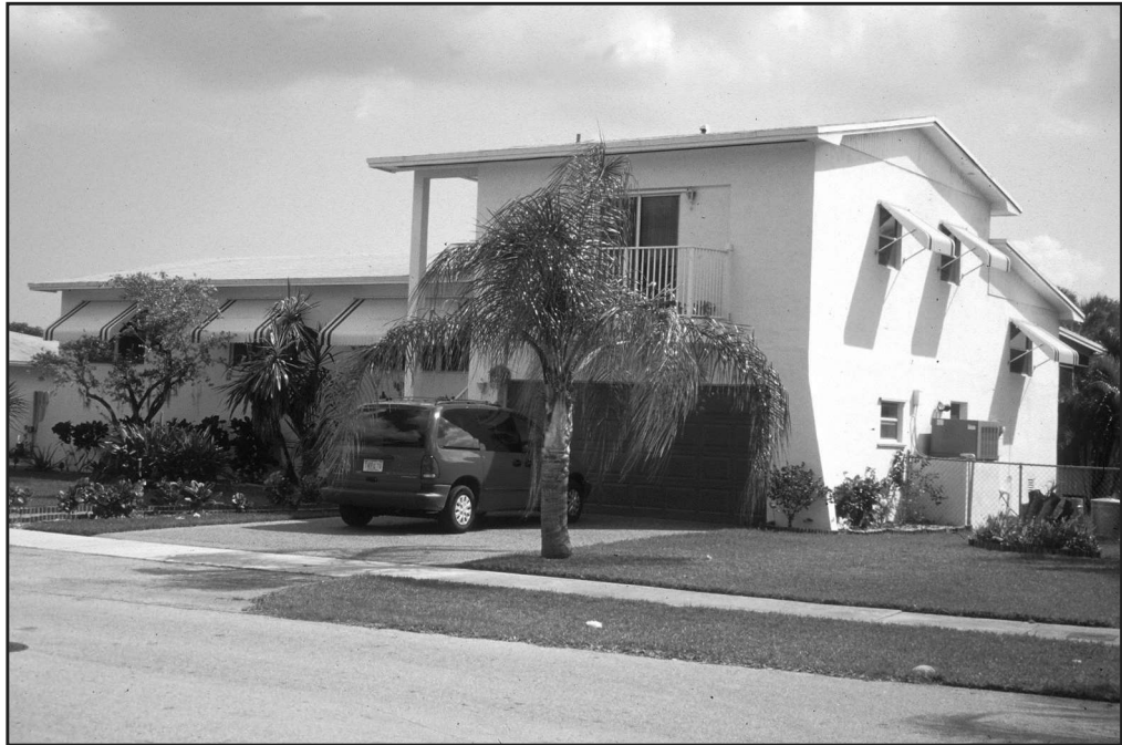
Figure 72 The completed house is compliant with local floodplain management requirements, is more resistant to flood damage, and provides additional living area above the flood level.
