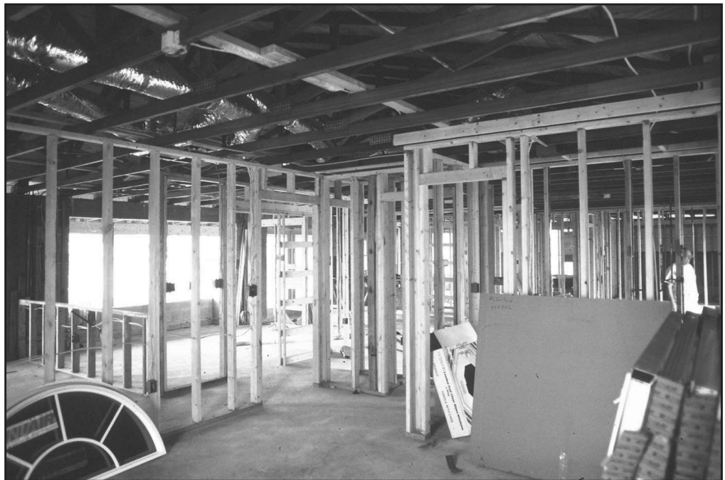
Figure 30 Interior partition walls and utilities are added.
