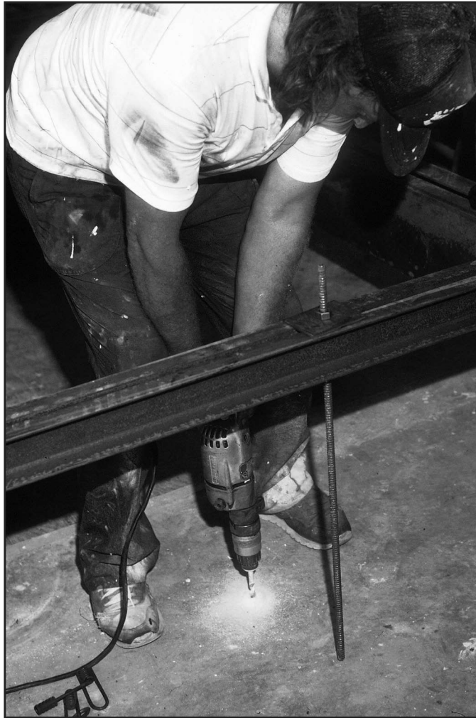
Figure 77 ... install anchors ...
