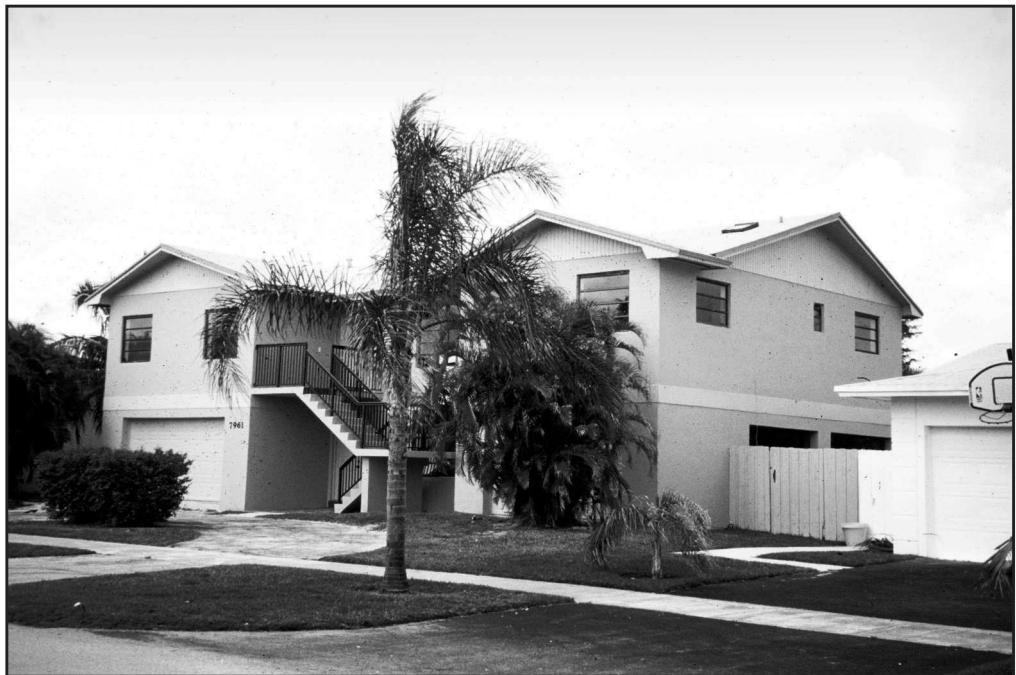
Figure 85 The completed house, with lower-level space for parking and storage and upper- level living space, looks as if it were originally designed and built as a two- story structure.
