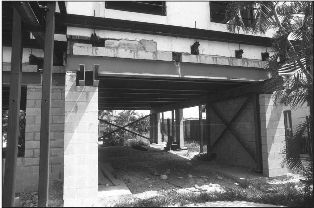
Figure 84 ... and used to build the lower-level walls.
