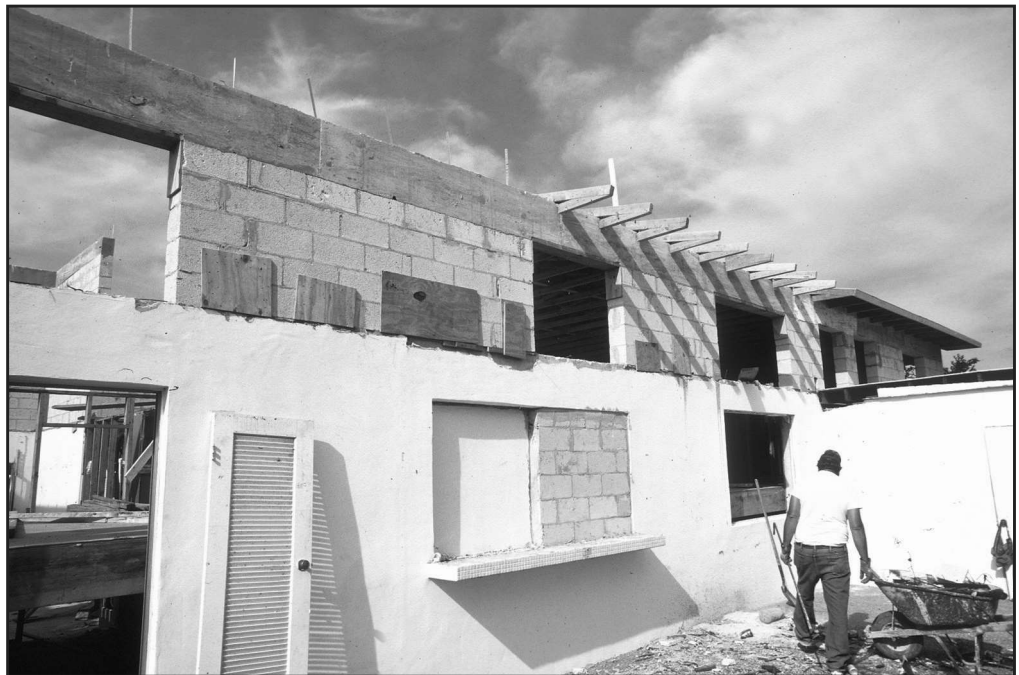
Figure 67 The extended first-story walls.
